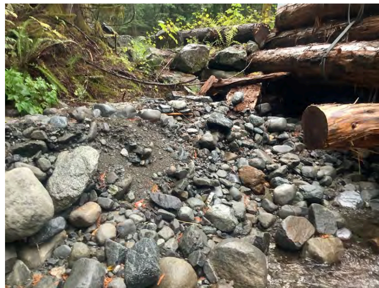
Left Bank Abutment when facing downstream
