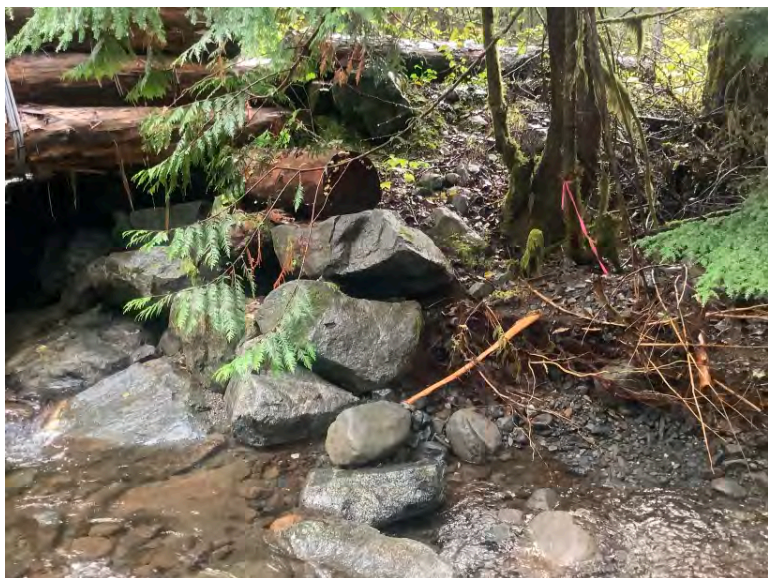
Left Bank Abutment when facing downstream
