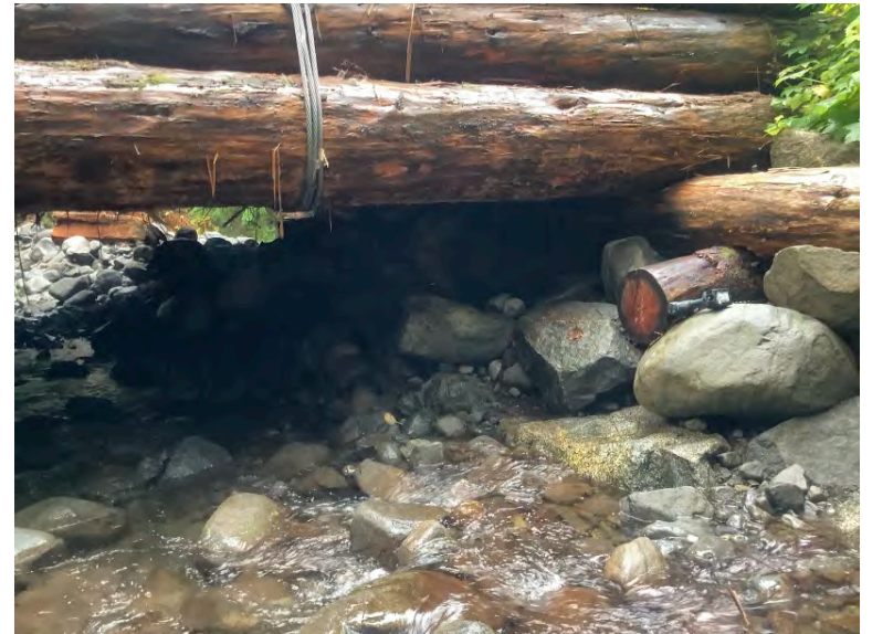
Right Bank Abutment when facing downstream
