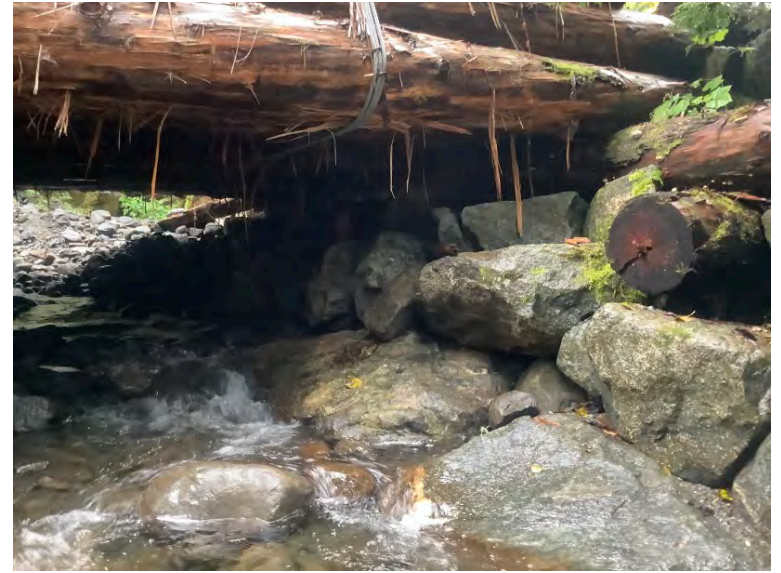
Left Bank Abutment when facing downstream
